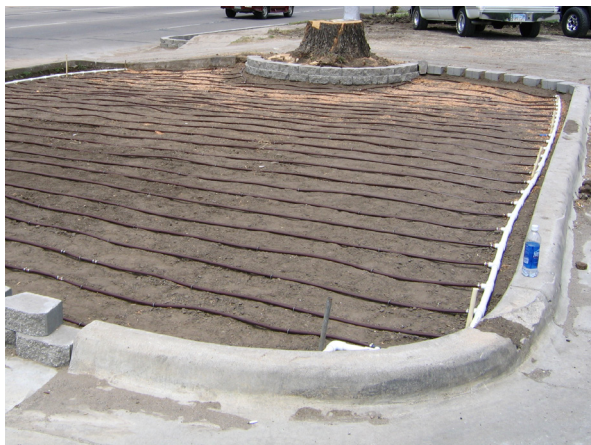
Low Output Device, Subterranean Drip Tubing
