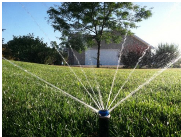
Low Output Device, Stream Rotor
